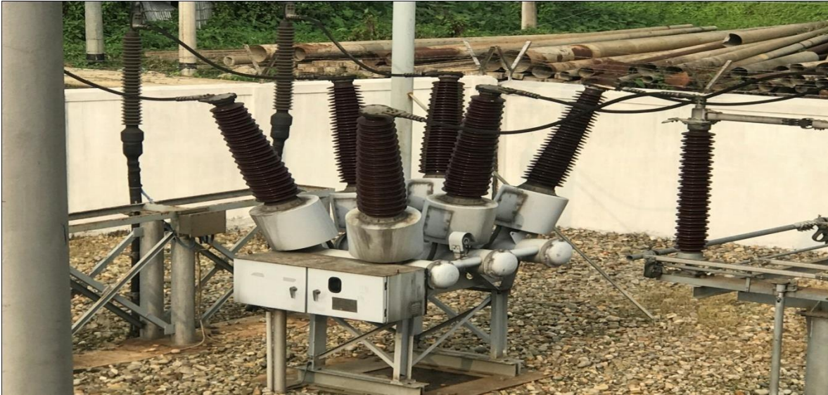
Figure 3.5: SF 6 Circuit Breaker
