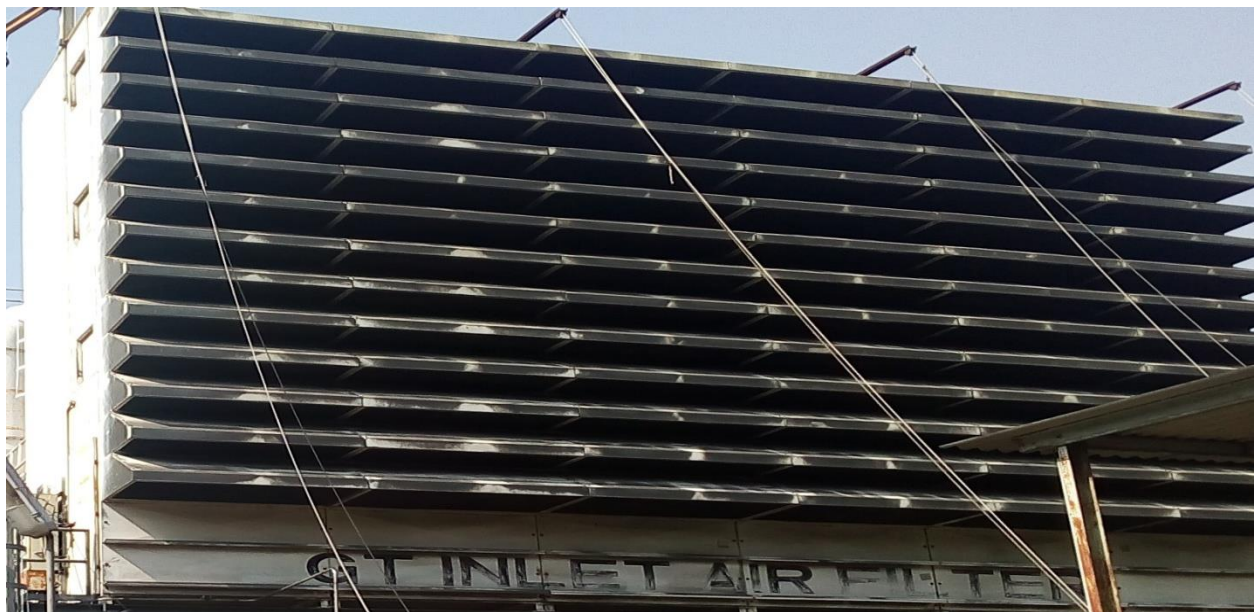
Figure 4.1: Air Intake Filter
