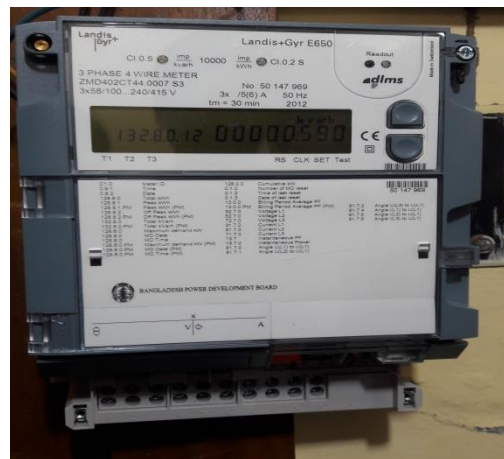
Figure 5.12: Single phase meter (digital) [2]
