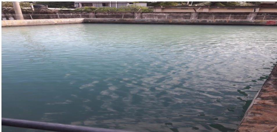
Figure 2.5: Demi water storage tank at Katakhal power plant [2]
