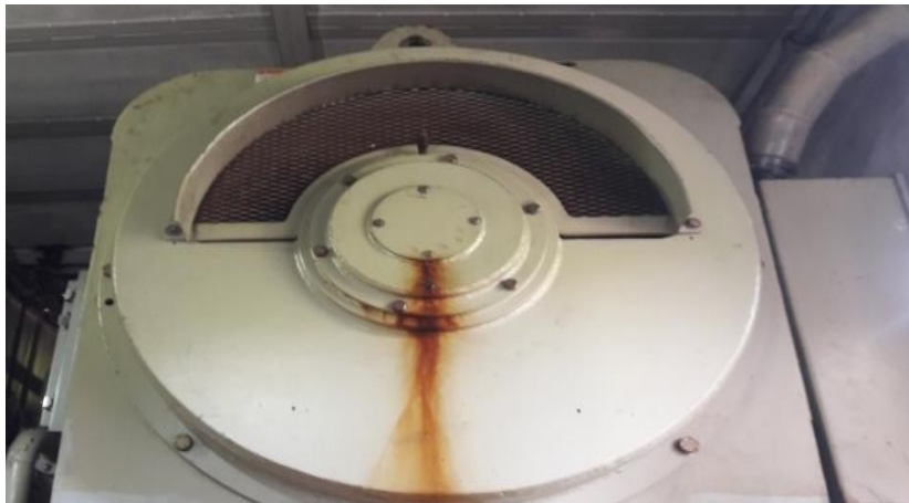
Figure 3.2: Front view of 100 MW generator at Baghabari power plant [2]
