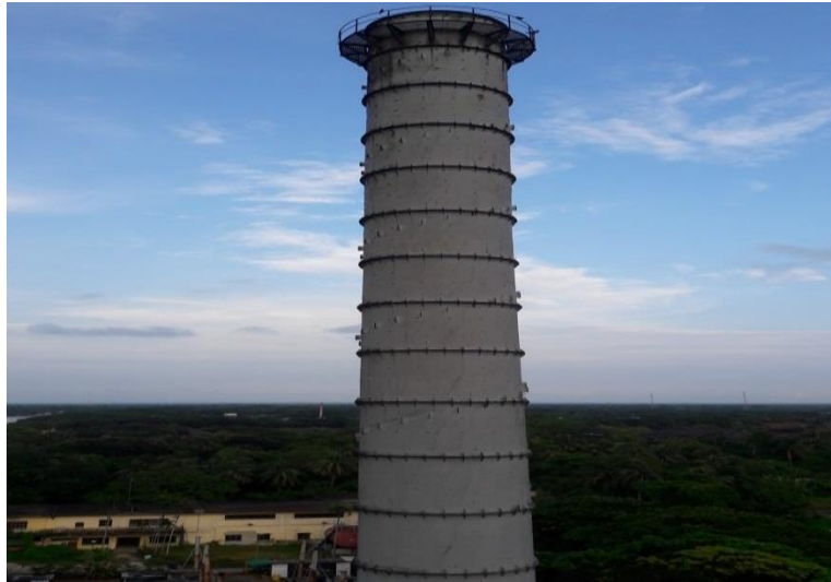
Figure 4.5: The structure of chimney at Khulna power plant [2]
