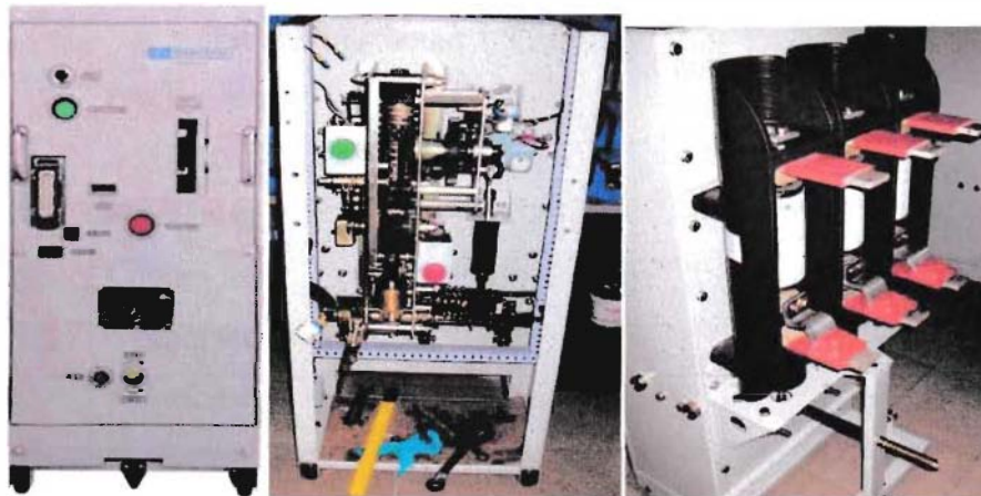
Figure -: Indoor type VCB driving Box front view; internal view; VCB Interrupter
