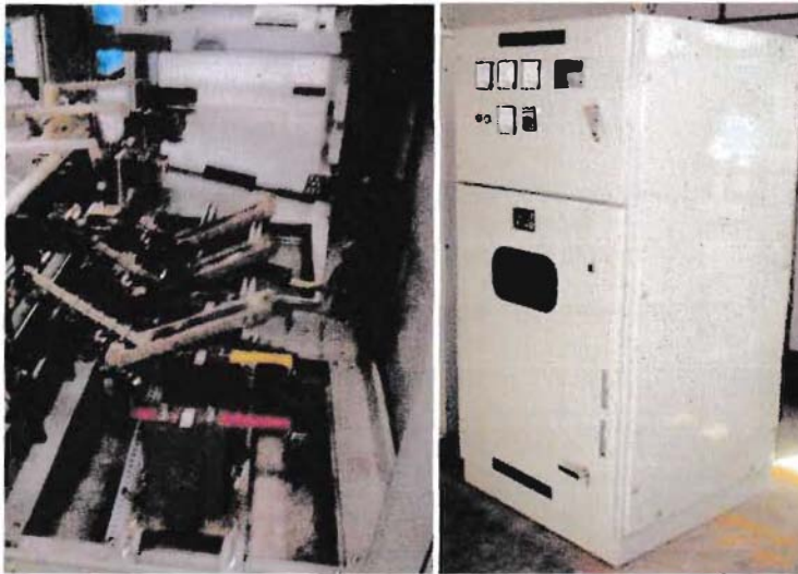
Figure -: Internal and external view of LBS
