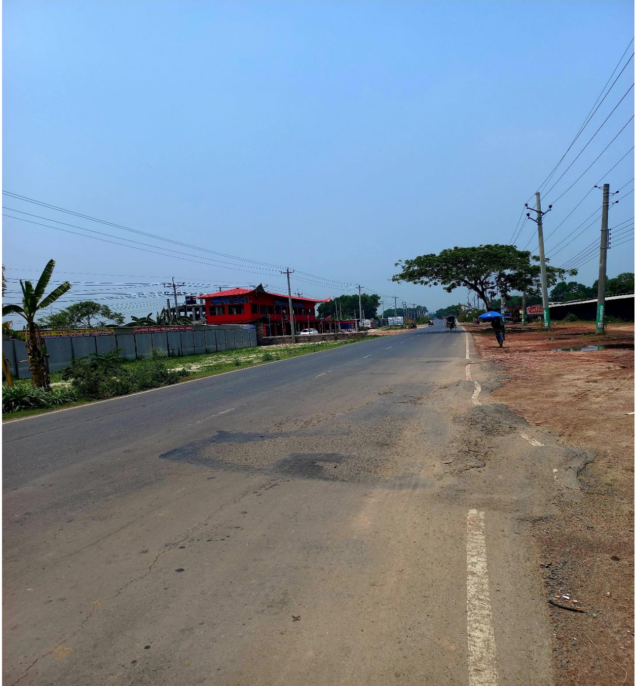
Figure: Real picture of N808 (this is an actual flexible pavement)
