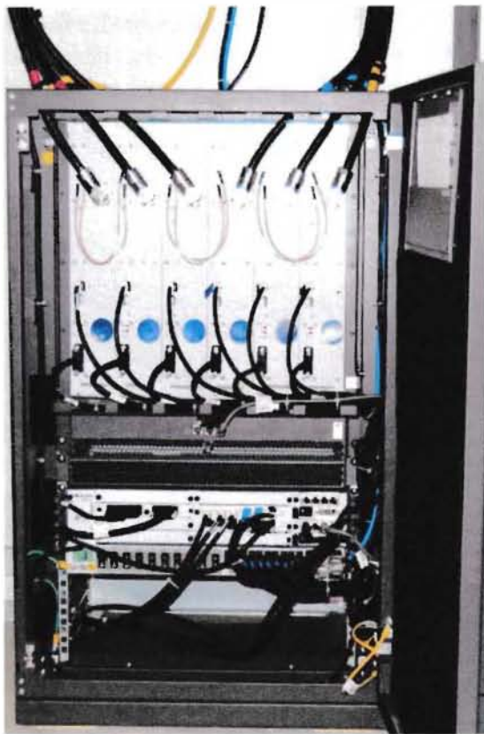
Figure 2-5: BTS 3900 Indoor view
