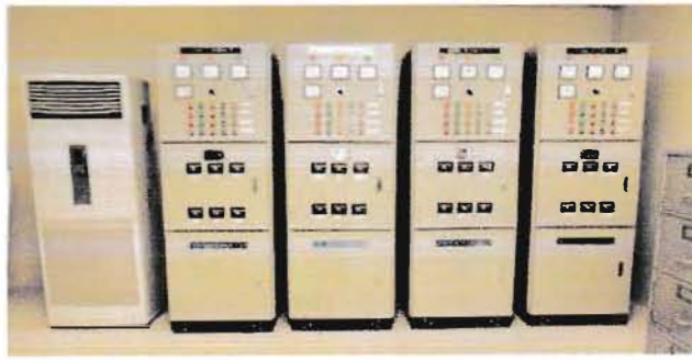
Figure 27: LT metering panel ( www.energypac.com )
