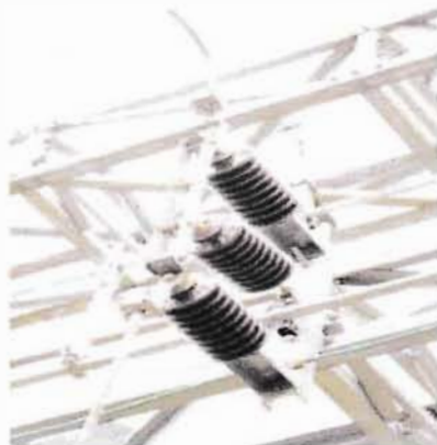
Figure 46: Center Breaker Isolator ( www.energypac.com )
