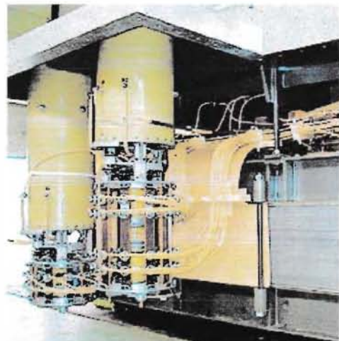
Figure 24: Block Diagram of tap changer and physical view of Tap changer ( www.thefullwiki.org )
