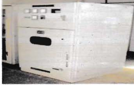
Figure 31: Load Break Switch (www.energypac.com)
