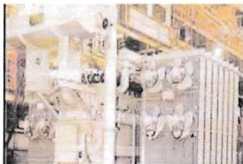
Figure 22: Oil Immersed Air Blast - Type ONAF (www.electrical-engineering-portal.com)
