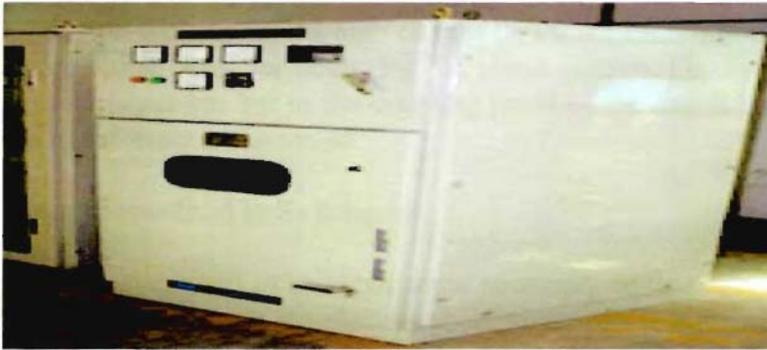
Fig 23: Load Break Switch. [7]
