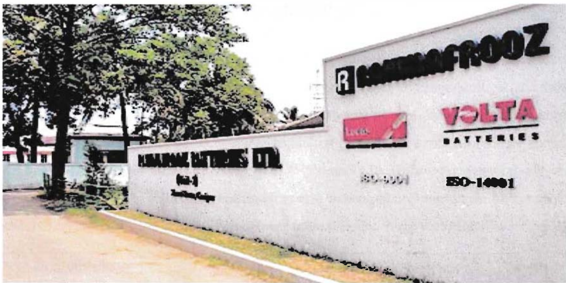
Figure 1.2.a: Main entrance at Saver Plant
