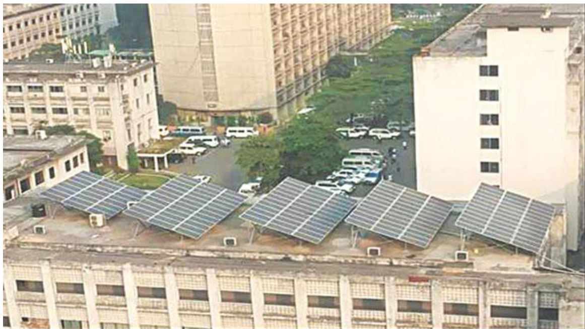
Figure 1.1: Image of DPDC's Rooftop Solar Power Project at Bangladesh Secretariat
