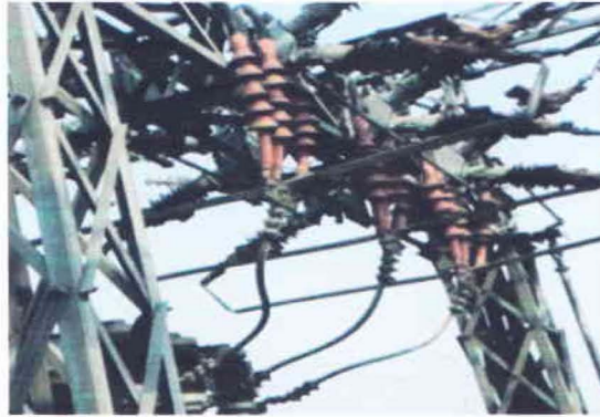
Figure 3.15: Strain Insulation used for High Range
