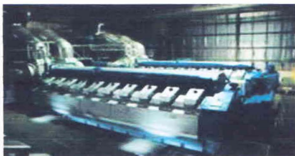
Figure 2.2: Generators of Summit Power Limited
