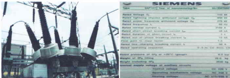
Figure 3.10 SF 6 Circuit Breaker of used for High Voltage Protection
