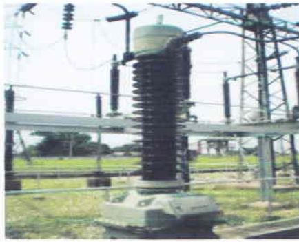
Figure 3.3: Potential Transformer
