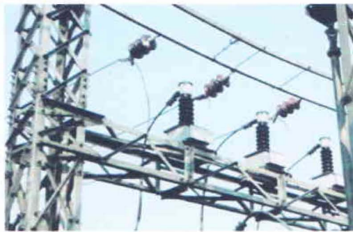
Figure 3.14: Suspension Type Insulator used for Medium Range
