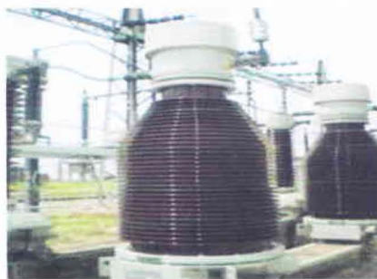
Figure 3.2: Current transformer
