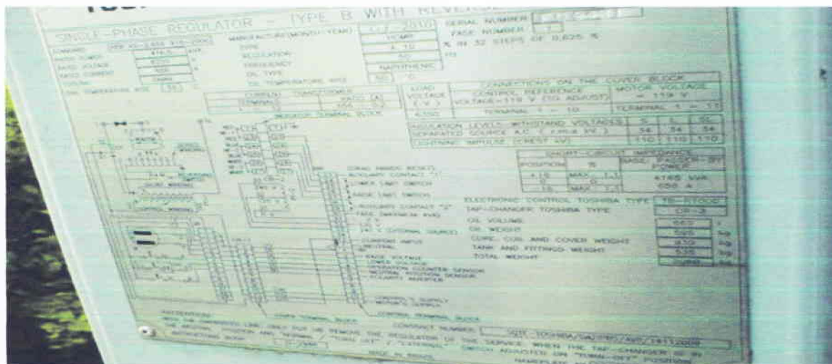
Figure 3.22: Nameplate of the Transformer
