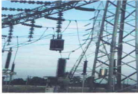
Figure 3.18: Wave Trap used for Communication
