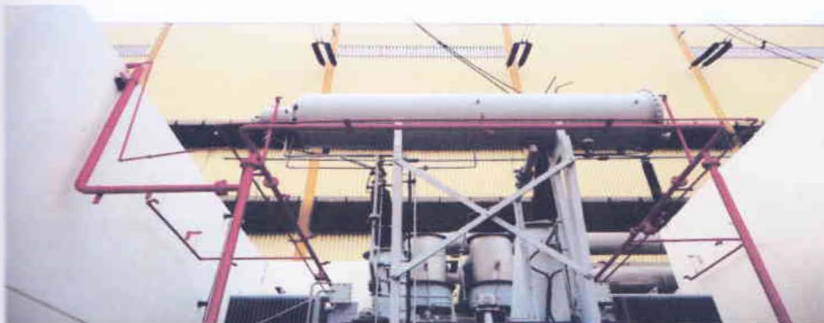
Figure 2.7: Step-up Transformer
