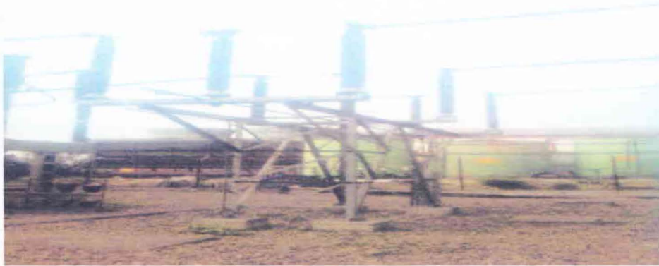
Figure 2.12: Isolators used in APSCCL
