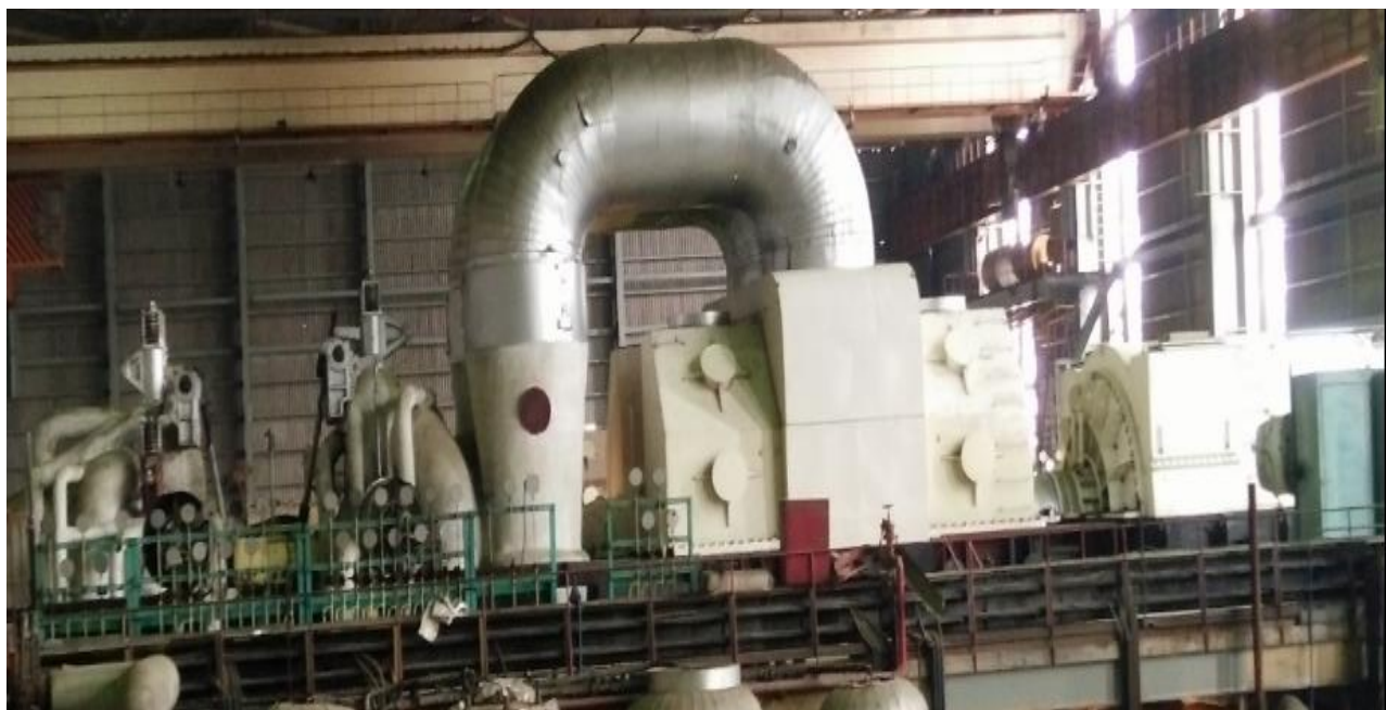
Figure 4.6: HPC, IPC and LPC of unit-4 at GPS.
