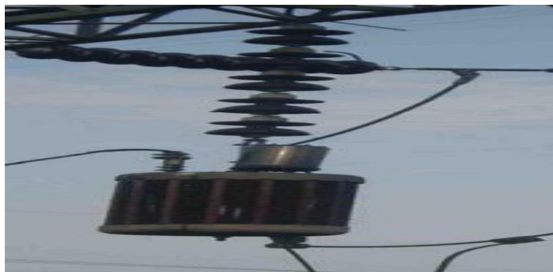
Figure 6.13: Wave trapper at GPS.
