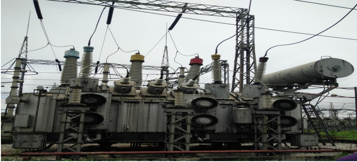
Figure 6.4: Auxiliary transformer.
