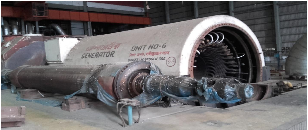
Figure 5.2: Stator and rotor at GPS (unit-6).
