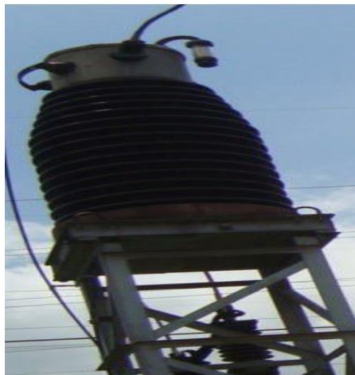
Figure 6.6 : Current transformer (CT).
