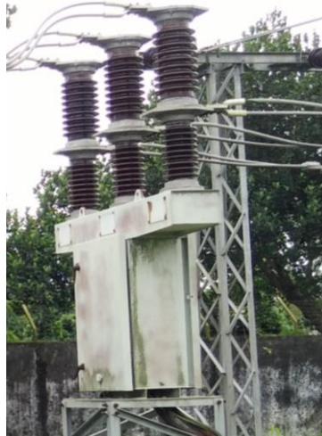
Figure 6.18: Vacuum circuit breaker.
