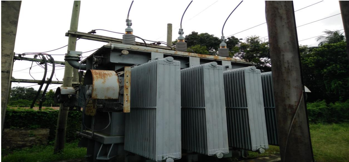
Figure 6.5: Coupling transformer.
