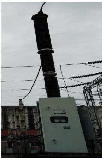
Figure 6.17: SF 6 circuit breaker.
