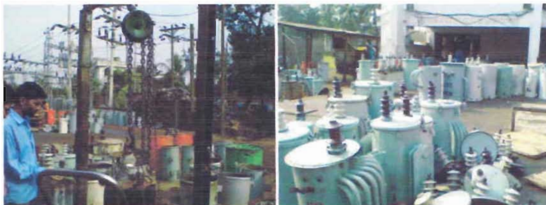
Figure 5.1: Repairing Transformer at PBS-1
