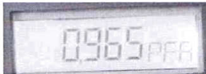
Figure 4.3 : Power factor cell of 33 KV feeder panel
