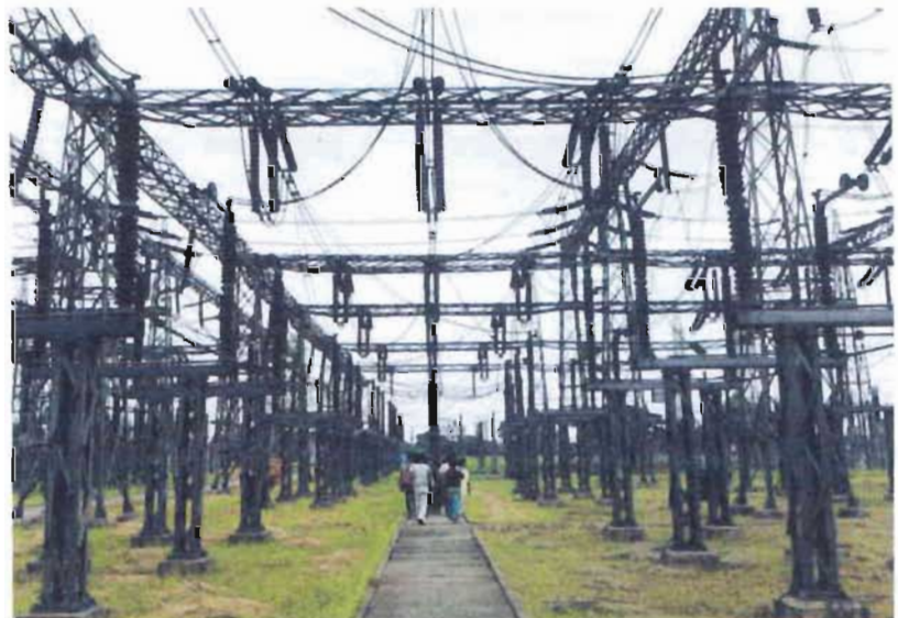
Figure 5.4: 230KV Busbar arrangement system of APSCS
