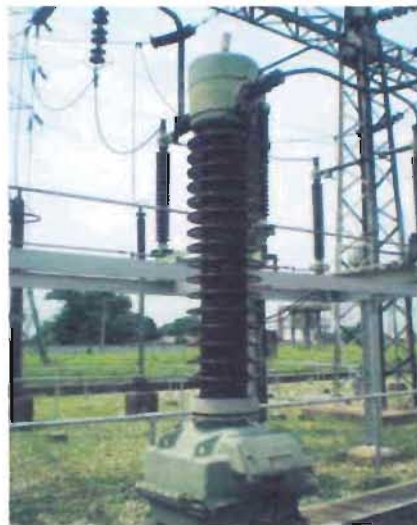
Figure 5.3: Conceptual Picture of a Voltage Transformer of 132KV line.
