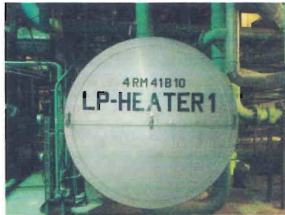
Figure 2.11: LP heater of steam power plant of APSCL
