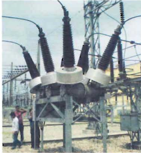
Figure 5.7: Picture of SF6 Circuit Breaker
