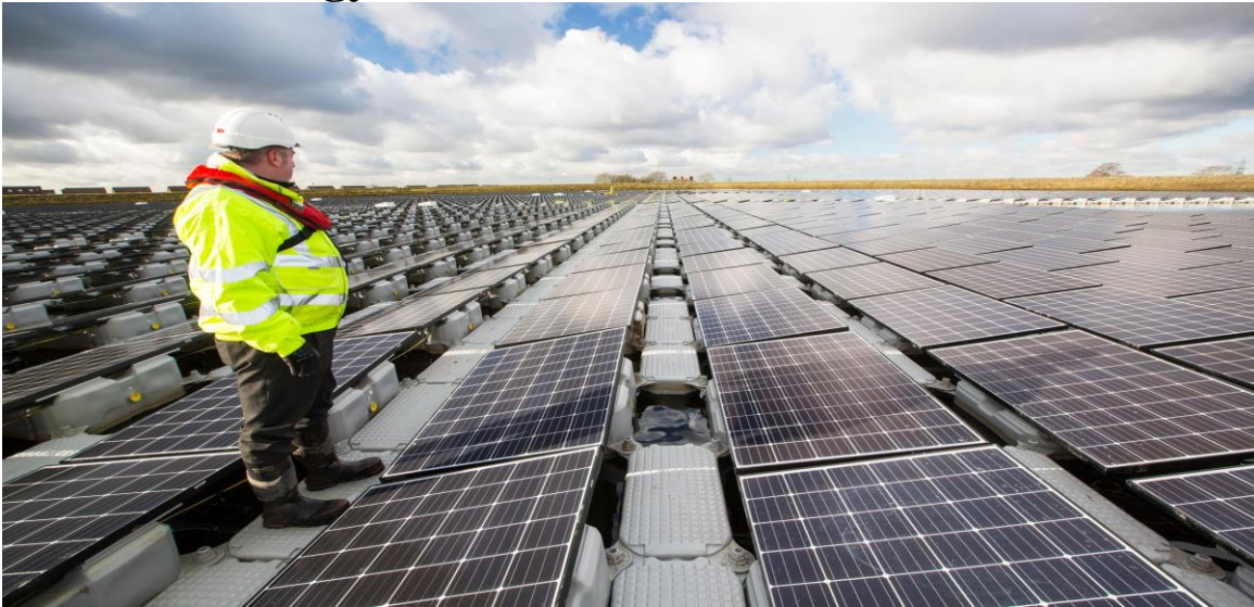
Fig.2.1 The Floating solar farm on Godley Reservoir near Manchester, UK.
