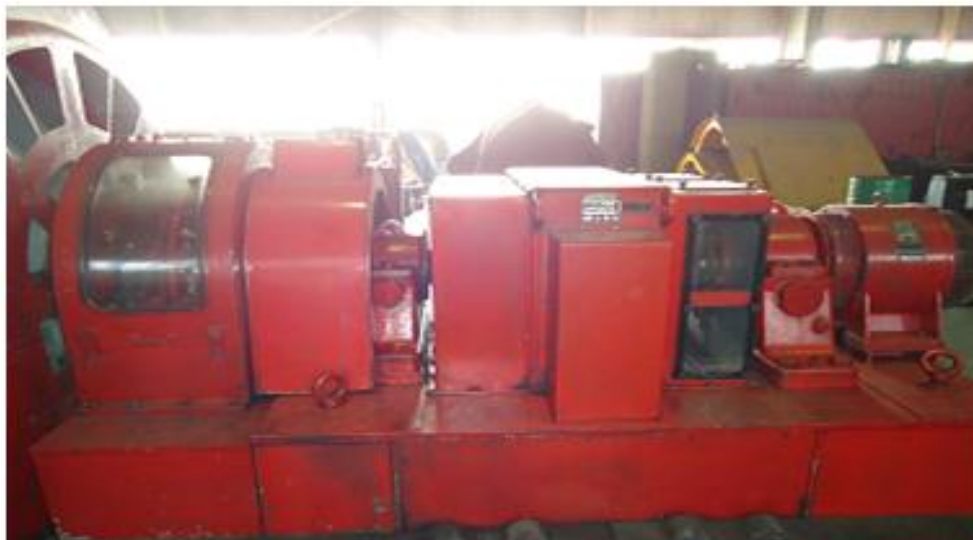
Figure 3.2: Excitation system of unit 2.
