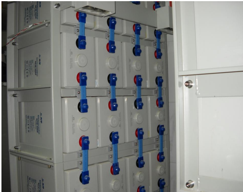
Fig 6.4: A unit dry cells which is used in BTS room
