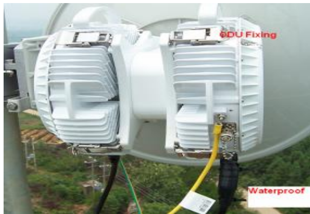
Fig3.5: ODU with antennas
