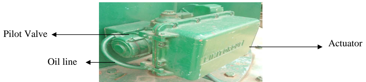
Figure 5.1: Hydraulic Actuator and Pilot valve.
