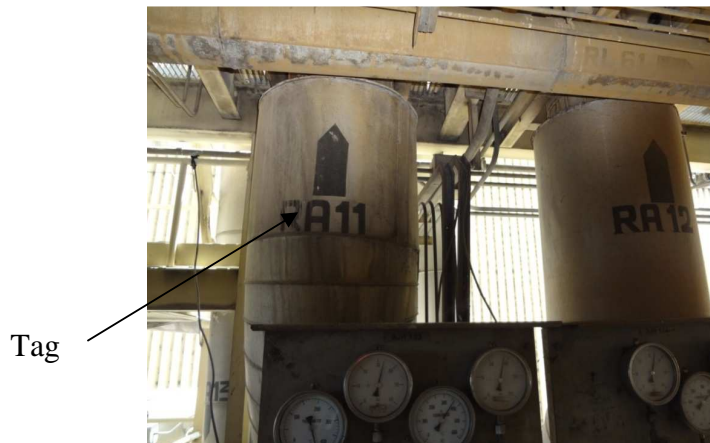
Figure 4.4: Pipe-lines of HP Bypass.
