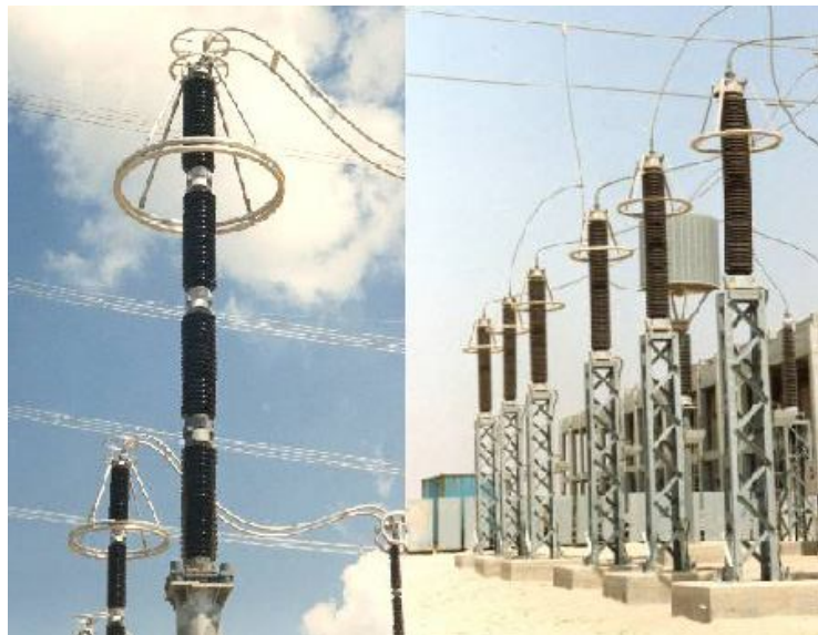
Figure 5.7: Lightning arrester, non linear resistor type
