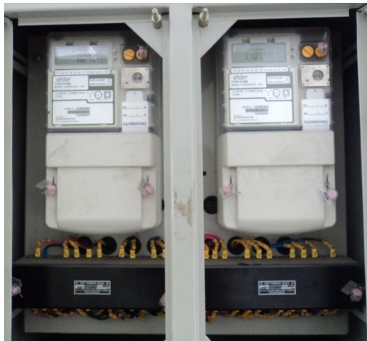
Figure 8.6: Energy meter to calculate the power flow
