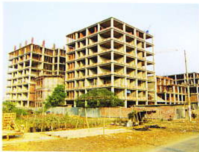
EWU Campus under Construction
