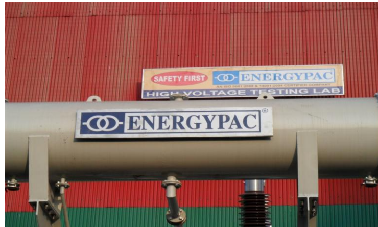
Figure 9: Conservator tank
