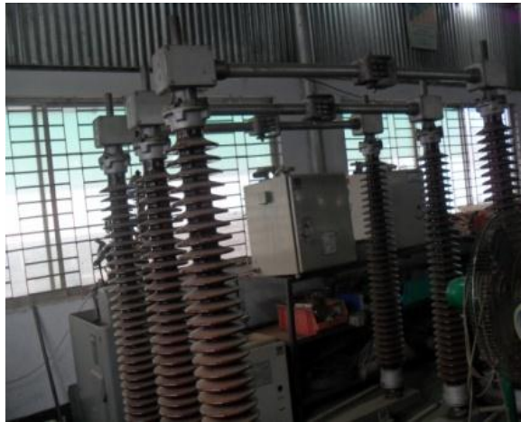
Figure 26 : Centre Break type Isolator
