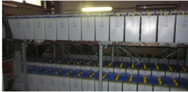
Figure 4.5: Series connected battery.
