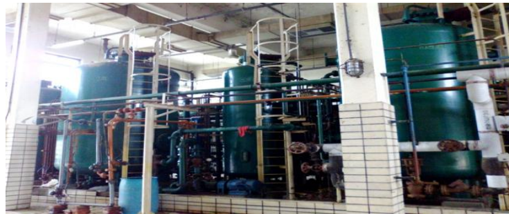
Figure 5.6: The Scavenger, Cation, Anion and Mixed bed filter.
