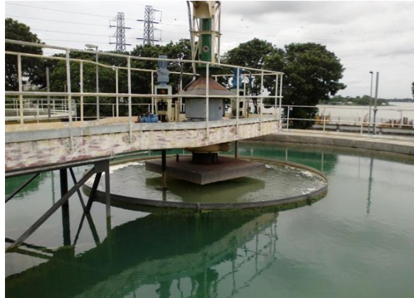
Figure 5.3: Water Treatment Plant.
