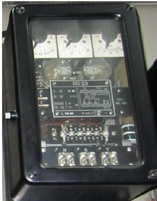
Figure 4.6: Generator Differential Relay.
