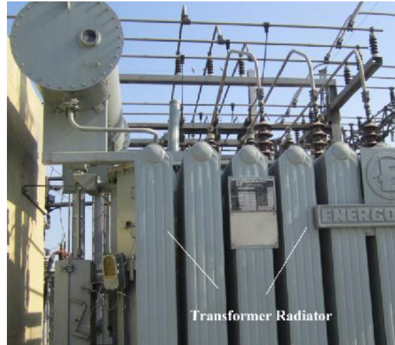
Figure 4.16: Transformer radiator for oil filled safe cooling.
