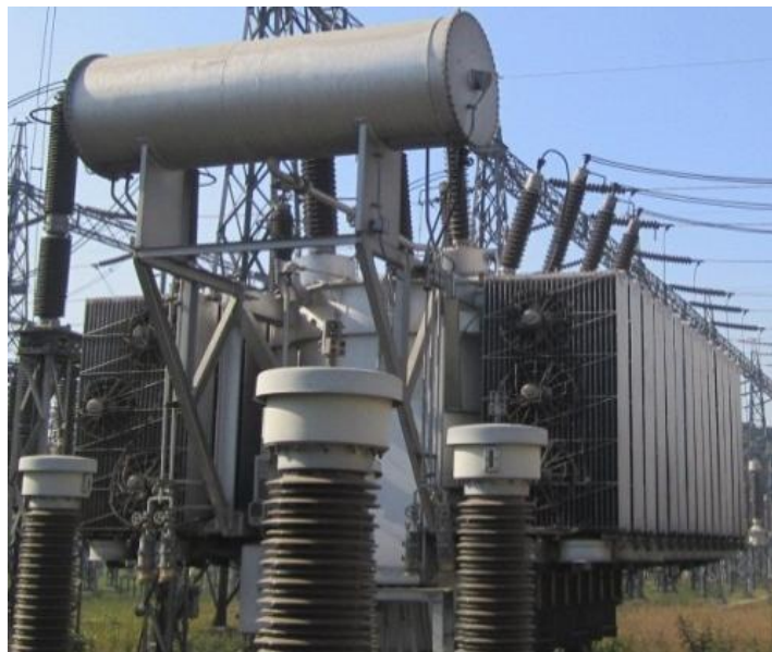
Figure 5.9: Intermediate potential transformer.
