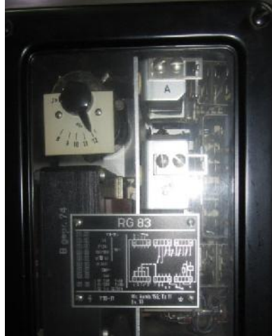
Figure 4.4: Negative phase sequence relay.
