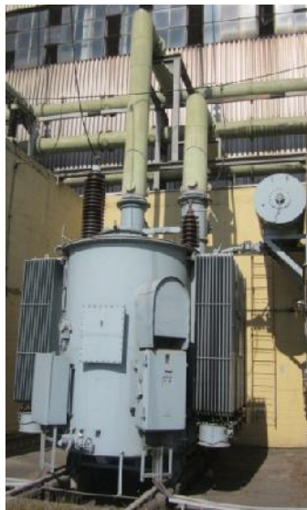
Figure 5.8: Single phase unit transformer.
