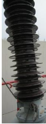
Figure 5.5: Bushing of power transformer.
