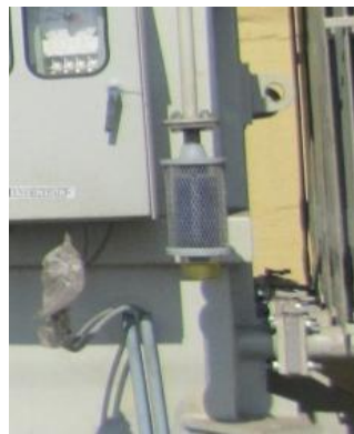
Figure 5.4: Breather of a power transformer.
