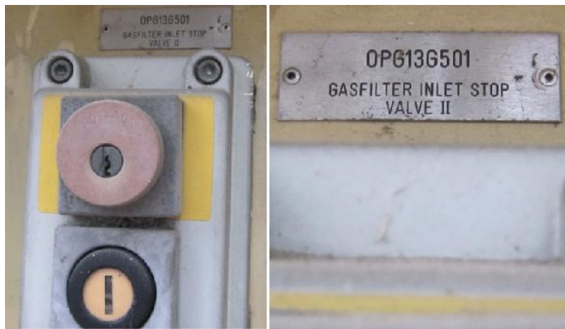
Figure 3.2: Gas filter inlet shut off valve.
