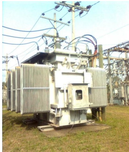
Figure 2.1: Power Transformer
