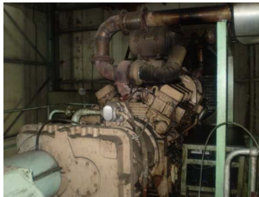
Figure 2.20: Diesel engine used in the gas turbine
