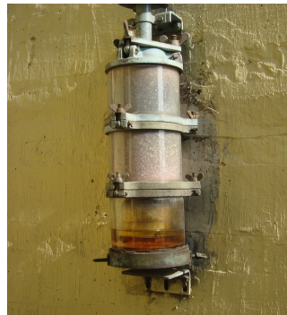
Figure 5.2: Transformer Breather
